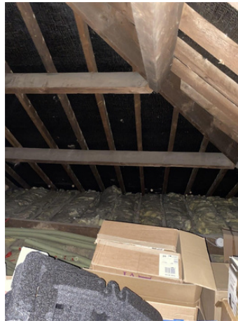
Date image taken: 2023:09:13 11:29:34 Latitude: 52° 36' 43" N Longitude: 1° 8' 7" W
